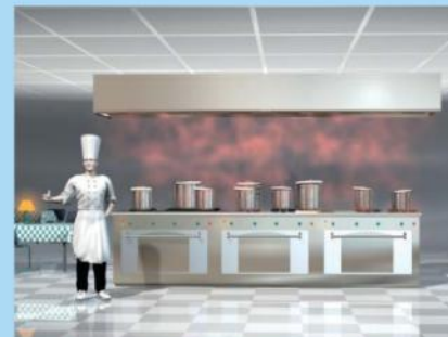
Picture 33. The hood should extend a minimum of 300 mm beyond the cooking equipment.
